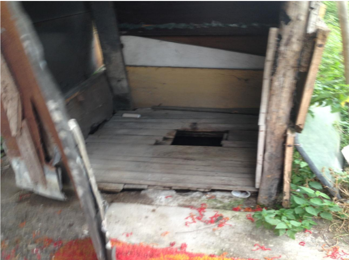
PHOTO [14] EXTERNAL TOILET.
