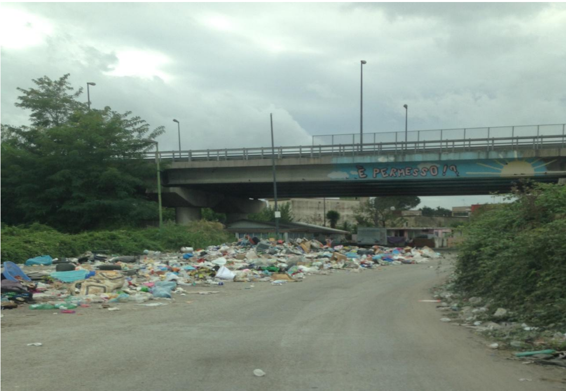
PHOTO [10] OVERPASSING ROAD AND RUBBISH.
