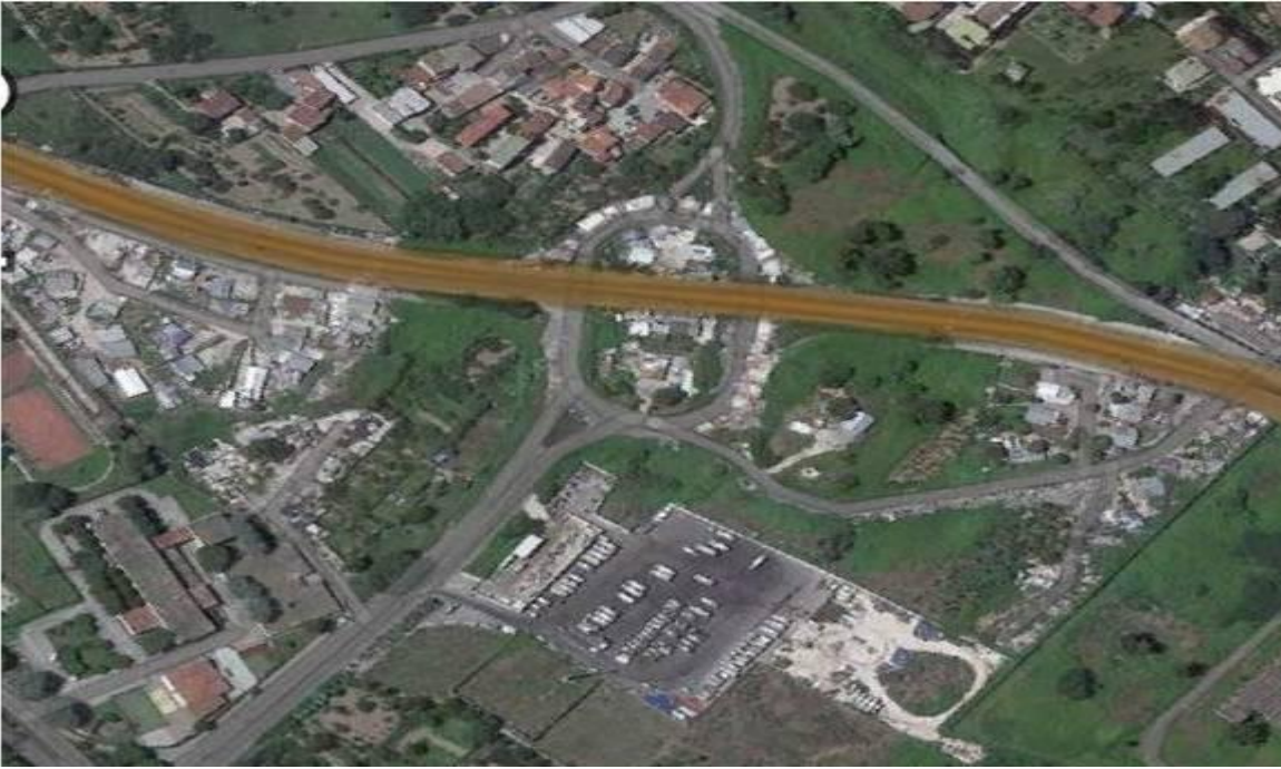
PHOTO [3] THE " OLD CAMP", VIA CUPA PERILLO, SCAMPIA (AERIAL VIEW) SOURCE: GOOGLE MAPS WEBSITE.
