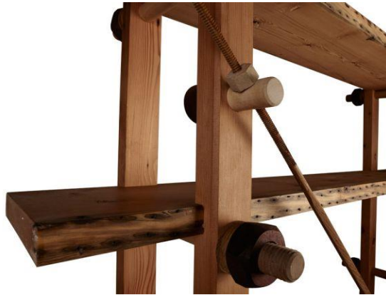
Figure 63 – Instead of commercially available joining methods, the Fenwick Ladder has been made by utilising a series of handmade wooden nuts and bolts
