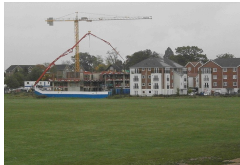
Figure 4-6: Playing field and construction site.
