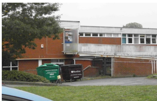
Figure 1-6: Entrance into E2E. View from inside of car passing through gate entrance.
