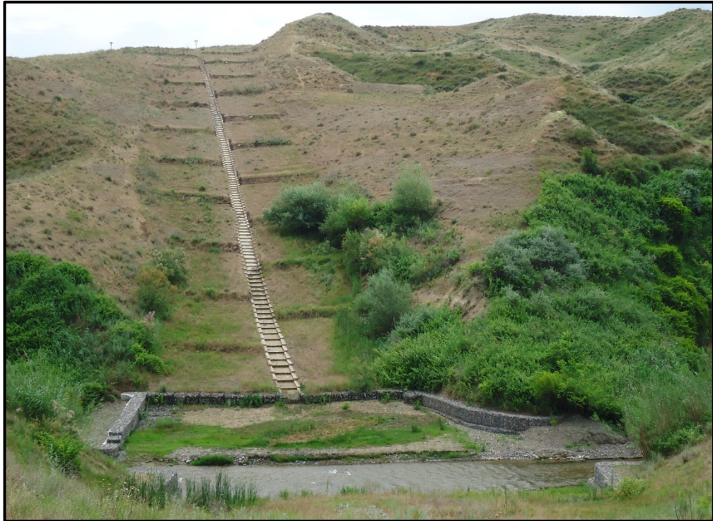
Figure 5.4 – Stone Waterway and Diversion Berms (Hassan Su - Azerbaijan)
