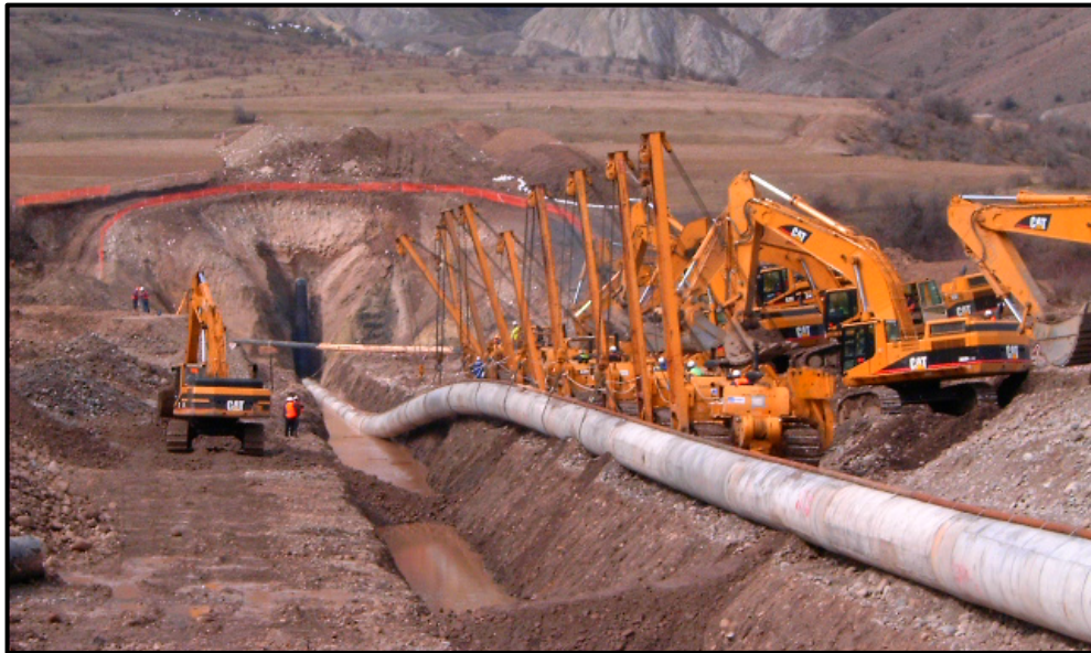
Figure 1.14 – Pipeline Lower and Lay (Georgia)
