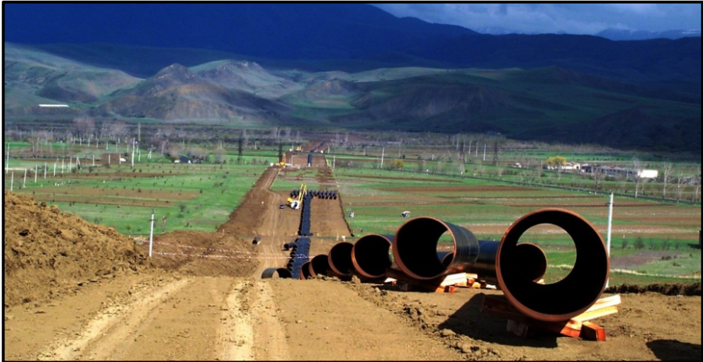
Figure 1.9 – Pipe Stringing (Georgia)
