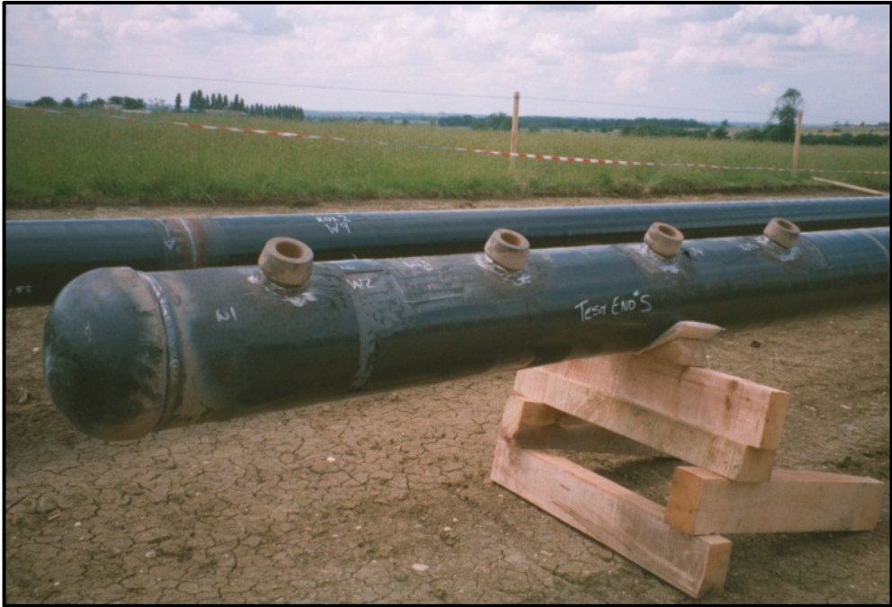
Figure 1.15 – Hydro Testing (UK)
