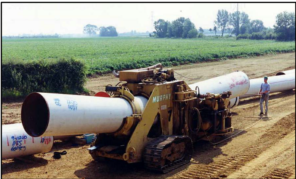
Figure 1.10 – Pipeline Bending (Georgia)
