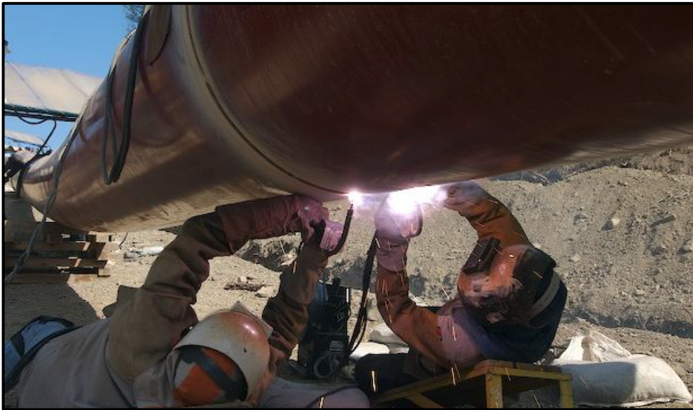
Figure 1.11 – Pipeline Welding (Canada) (CEPA, 2013)
