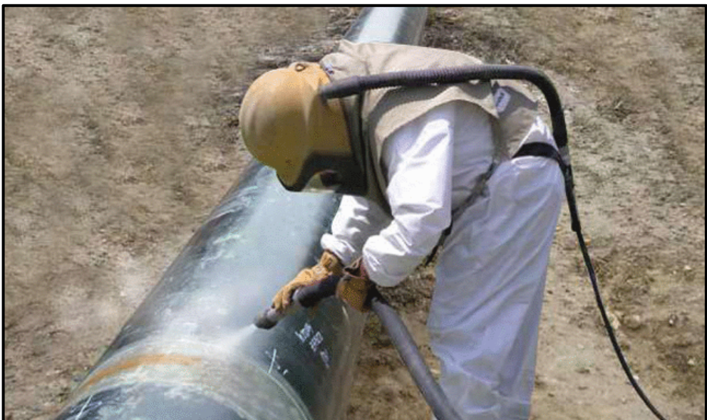
Figure 1.13 – Field Joint Coating (EPC, 2013)
