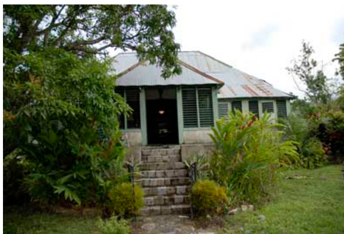
Figure One: Rock River Great House, is a typical penn style house with steps going on to the piazza, this house has the piazza enclosed with jealousies
