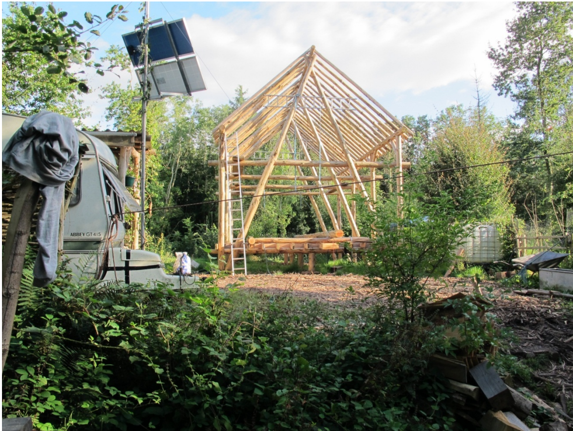
Figure 14: Green building by Paul Moreton in Moreton woods, Herefordshire, UK
