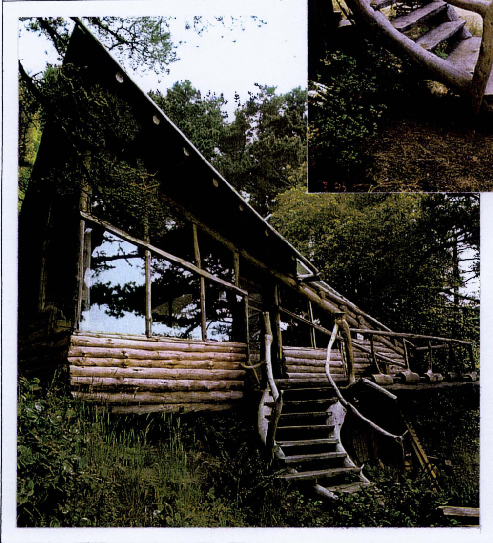
The 'Adirondack' tradition of the use of rustic timber in buildings, as in furniture, continues today. Note the use of such timbers for the veranda handrail supports and in the construction of the staircase of this forest cabin, built by a retired engineer in California, USA
