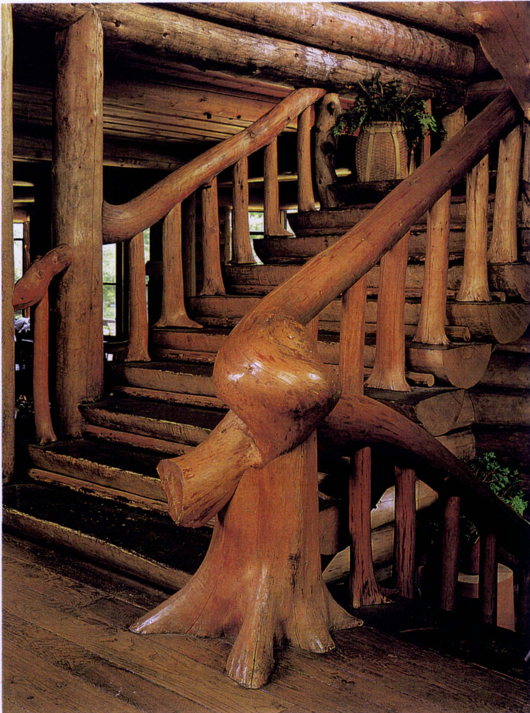
'Adirondack' staircase of peeled Spruce built in 1937 - 1938
