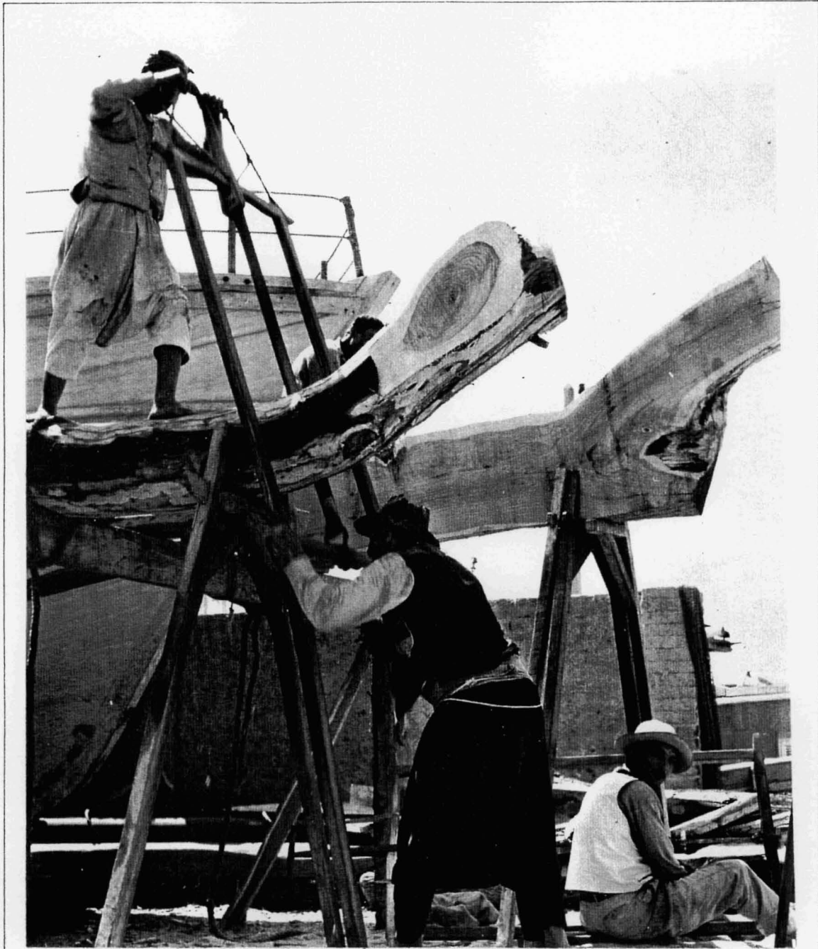
As in many countries, Egyptian boatbuilders take advantage of the naturally curving shapes to be found in timber
