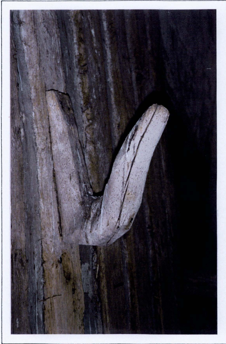
A natural timber fork used as a robust hook, seen in 1998 at Smallhythe Place, in Kent. Bought by the actress Ellen Terry in 1899, the cottage is now owned by The National Trust
