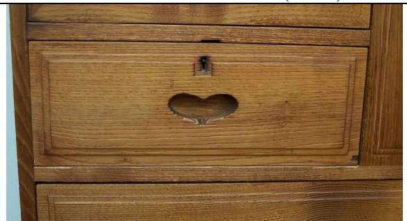
Fig. 2-25. 1904 '401' & '402' etc. suite handles. N.B. these were originally not polished but the colour of old brass. Drawer seals flush to front (author).
