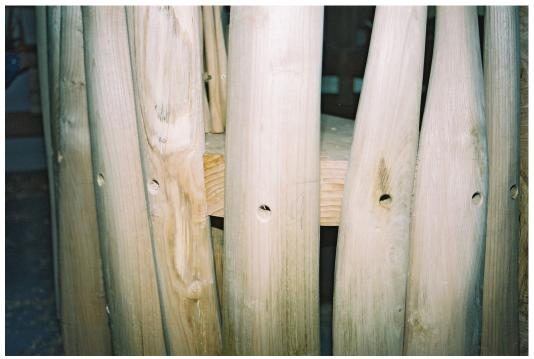
Fig 12. Reeds are positioned and pre-drilled
