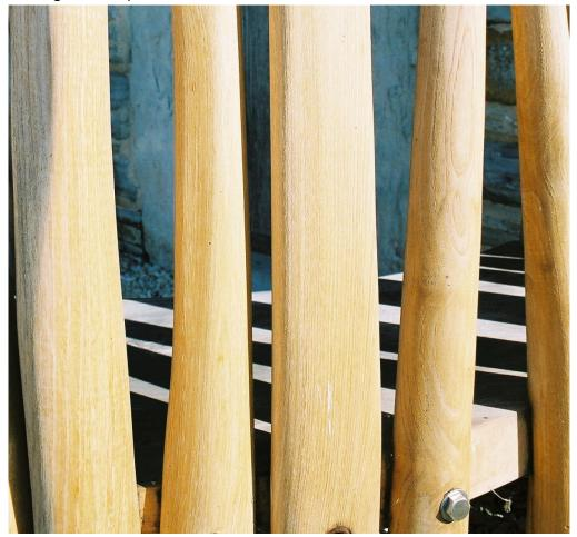
Fig 14d. The surfaces of these reeds were against the barn wall and therefore less exposed to the weather; no staining took place
