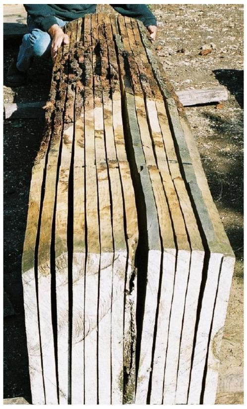
Fig 35b. The boards are arranged in their original sequence to ensure the grain and figure of each board can be matched. Each board is then numbered for identification
